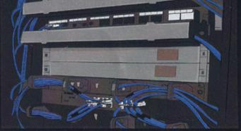
Snap the clips on the back of the panel into the holes on either side of the rack.
