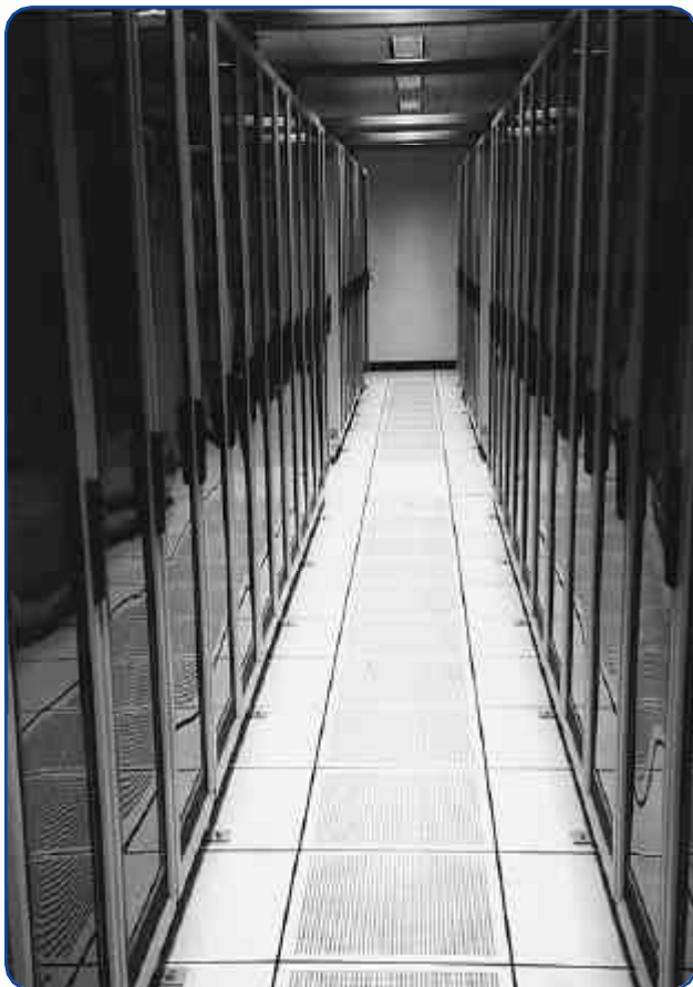
This cold aisle shows proper placement of perforated tiles on the intake side of IT equipment, but solid-front doors may be impeding the intake of cooling air. This site may experience problems as product heat densities rise.
